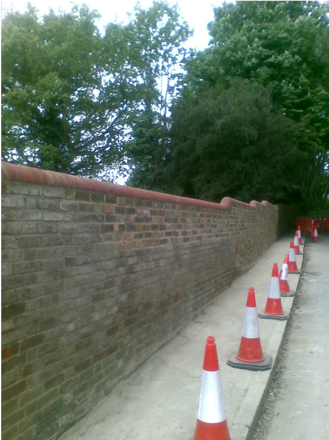
Boundary Road Wall Complete
